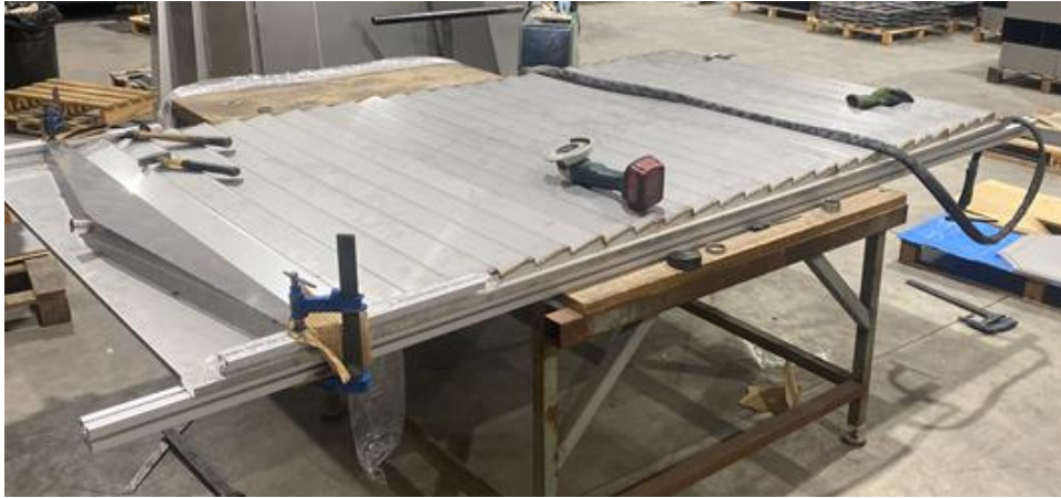
Figure 15: Image of the welding process for cascade component
