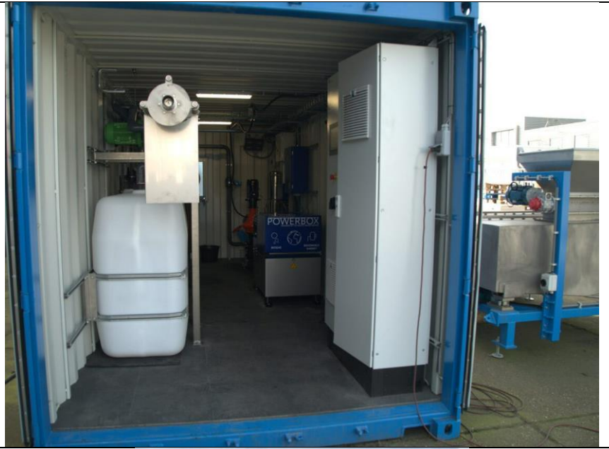
Installation of the electrical cabinet with the HMI screen
